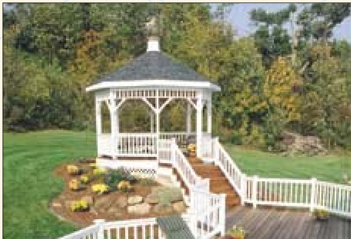
Romantic gazebo and deck. A nostalgic 12-foot diameter octagonal gazebo rests on a pod attached via a staircase from a deck addition. Gazebo elements, understructure and railings were painted a crisp white for extra eye appeal.
