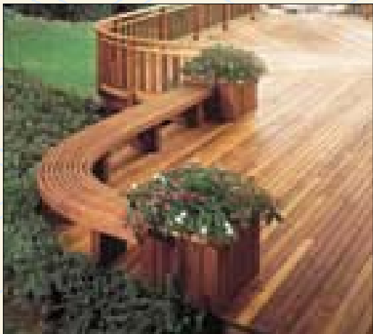
Curved deck with amenities. Handsome deck features an appealing curved bench flanked by built-in planters. The decking was installed in a herringbone pattern.
